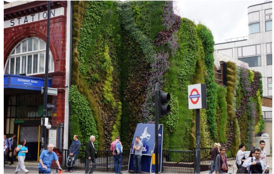
Biotecture Living Wall – Edgware Road London UK
